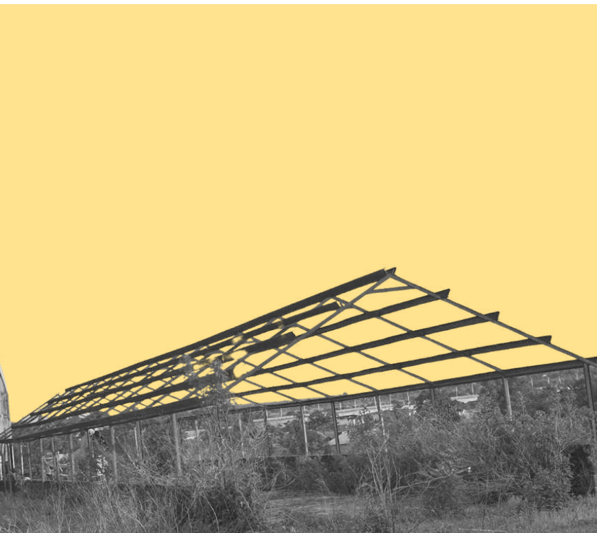
THE KATSINA-ALA YAM FLOUR PROCESSING COMPANY NEVER BECAME FULLY OPERATIONAL, AND ITS FACILITIES HAVE SINCE BEEN ABANDONED.
